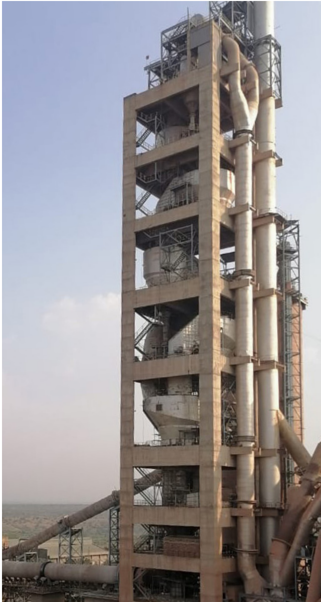
Pre-heater Building depicting Calciner and Cyclones
